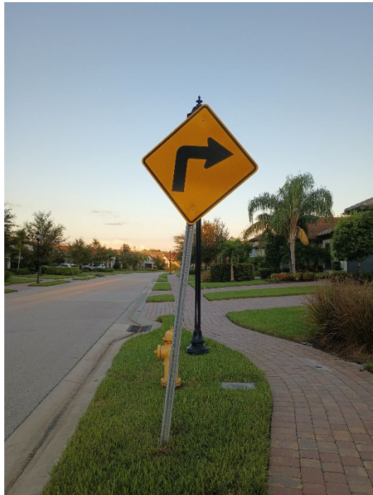
Right Bend Arrow Straighten Pole-Amaranda Court and Aviamar Circle. Temporary Sign-no concrete. In heavy rains ground gets soft.
