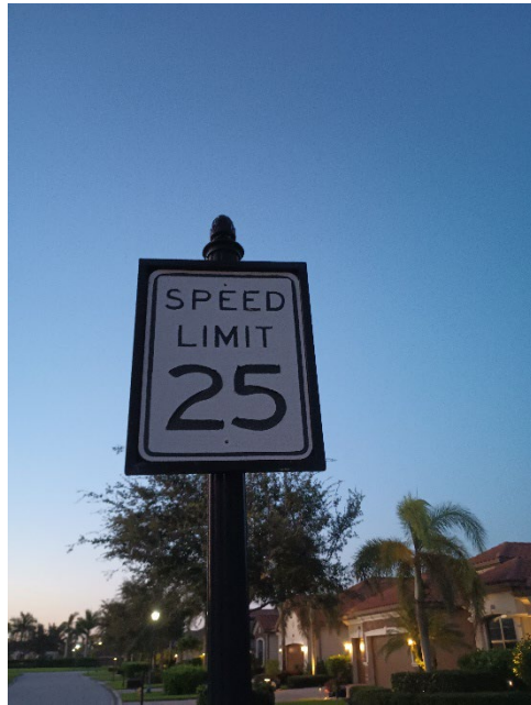
Carmini Court 25 MPH-Replace Sign Insert-Wrong Font?
