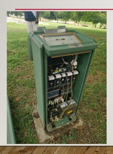
Satellite I-22 Sandpiper 3 – Identified electrical problem of insufficient power supply. Requested services of electrician.
